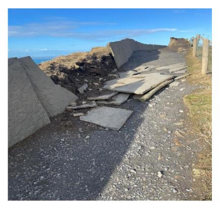
Figure 6-7: Damage to Liscannor Flagstones During Storm Eowyn
